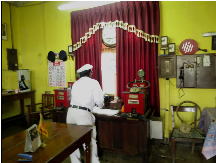
2010's-43: "Lock & Key" desk, Haputale station, a "Tablet" in place (and one sitting on the chair) – the system designed to allow only one train on a segment of track at one time (2016/05/07) [SANDRA DAWES].
