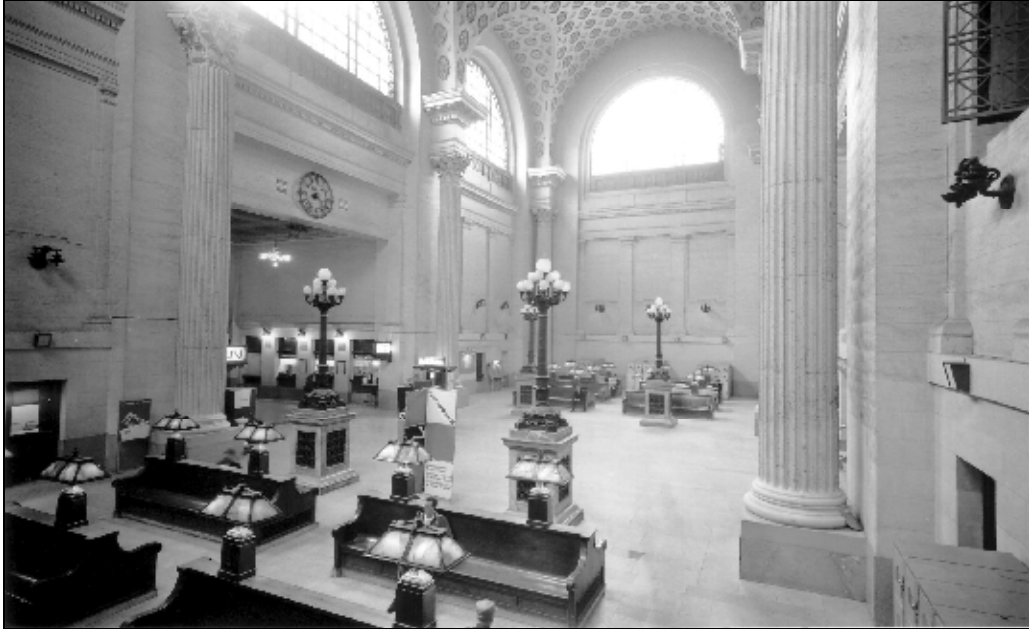
1950's-6: Ottawa Union Station's waiting area, with the passageway to ticket windows and concourse to the left (1966) [based on CLIFF BUCKMAN (LIBRARY & ARCHIVES CANADA/PA-155324)].
